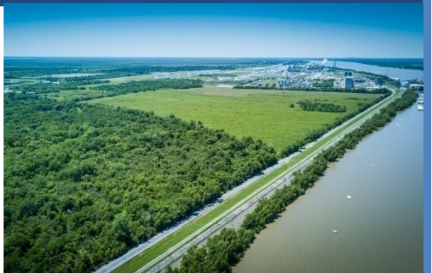
Fleeting Buoys In-Place
